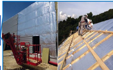
Thermal conductivity: 0.029 W/mK, Airtightness, q 50 : 0.17 m 3 /hm 2
