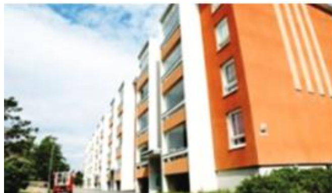
Figure 23 - Demo building Finland
