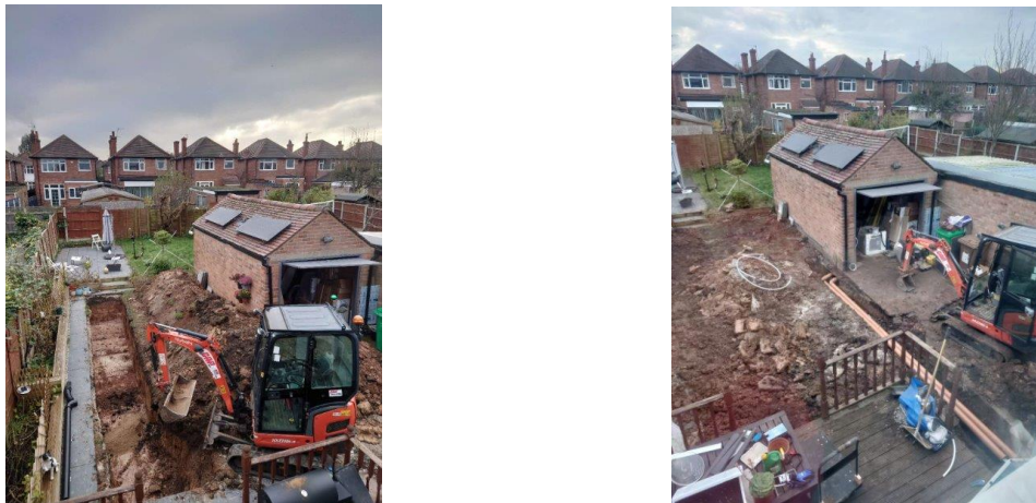
Figure 10 - Construction works at the UK demo building for the installation of the Ground Source heat pump
