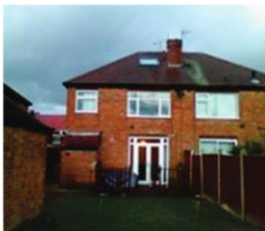
Figure 19 - Demo building UK
