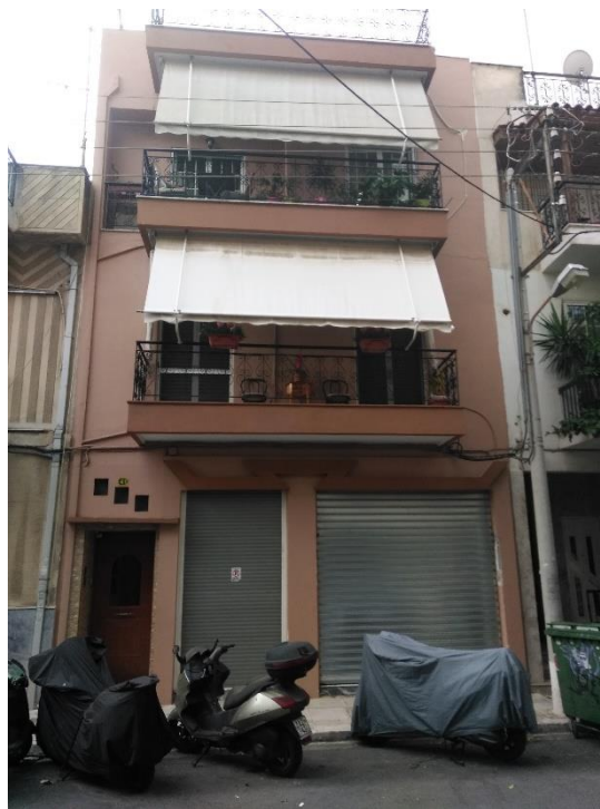
Figure 20 - Demo building Greece
