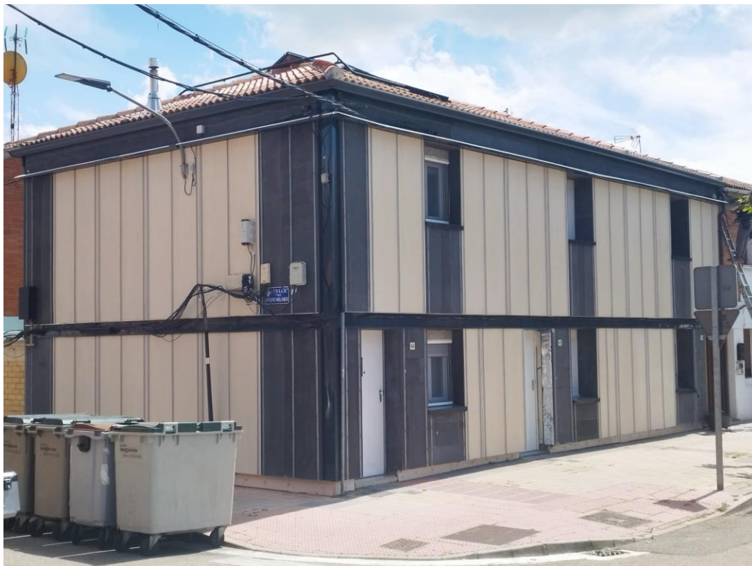
Figure 21 - Demo building Spain
