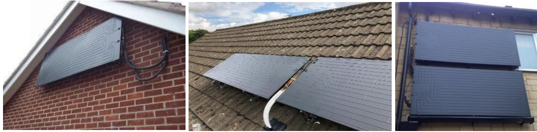
Figure 9 Installation positions of the thermodynamic panels
