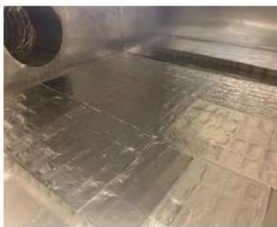
Figure 23 - A28 Blister panel in test box
