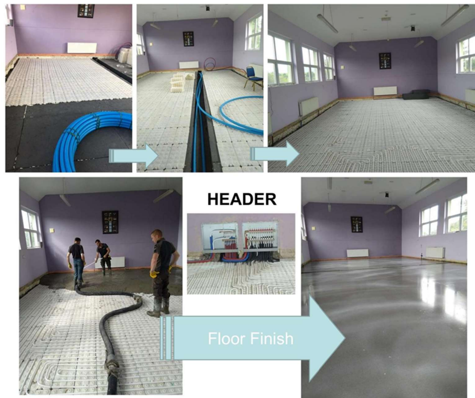
Figure 14 - Underfloor PCM installation
