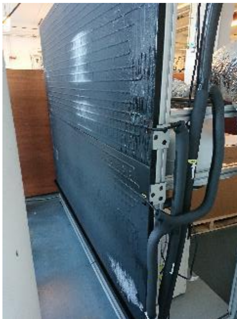
Fig. 12. Working sample of the thermodynamic panels
