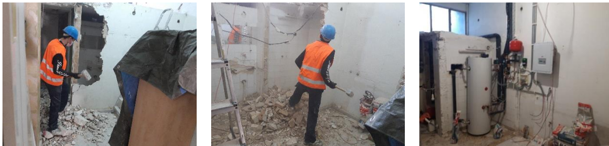
Figure 6 – Greek building: demolishing of WC to install the storage tank
