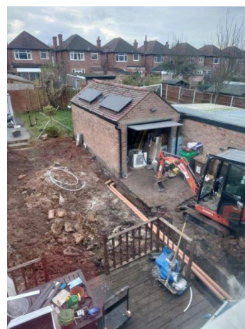
Figure 18 – Construction works at the UK demo building for the installation of the Ground Source heat pump
