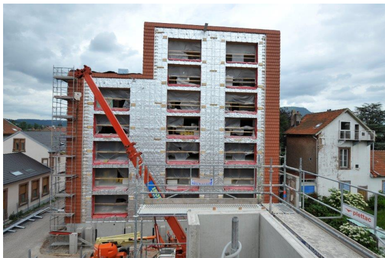
Figure 3 – SKYTECH Pro XL membrane installation in a high building
