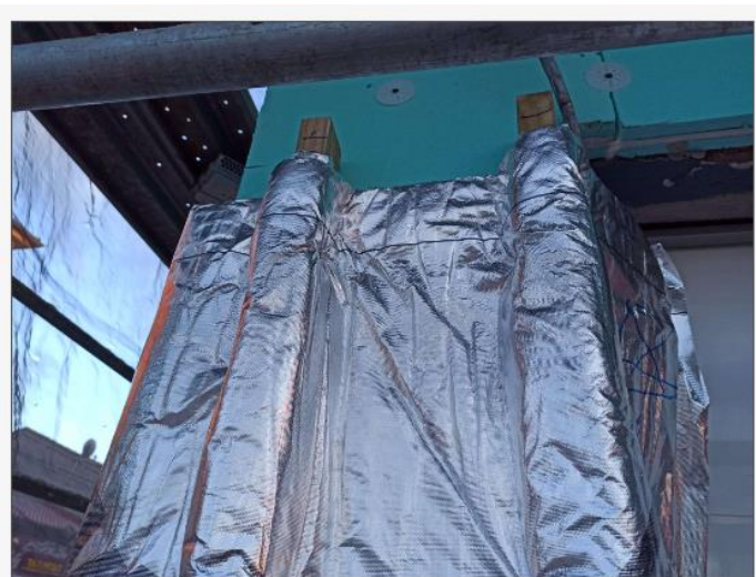
Figure 5 – Spanish building: challenges during installation of the 2cm membrane
