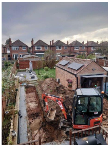
Figure 18 – Construction works at the UK demo building for the installation of the Ground Source heat pump
