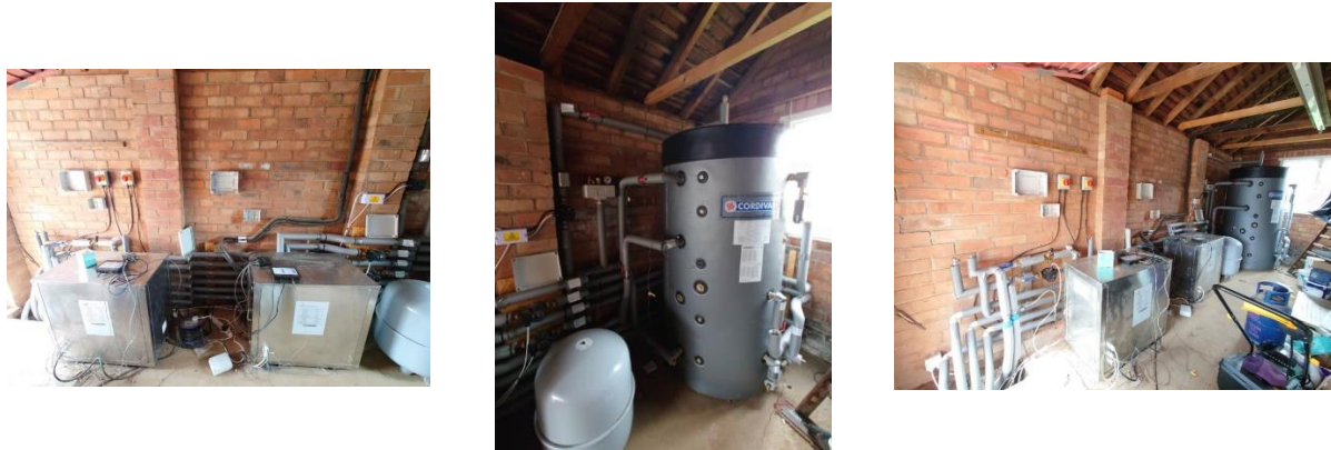
Figure 19 – Installation of the Solar assisted heat pump and the Ground source heat pump at the UK demo building
