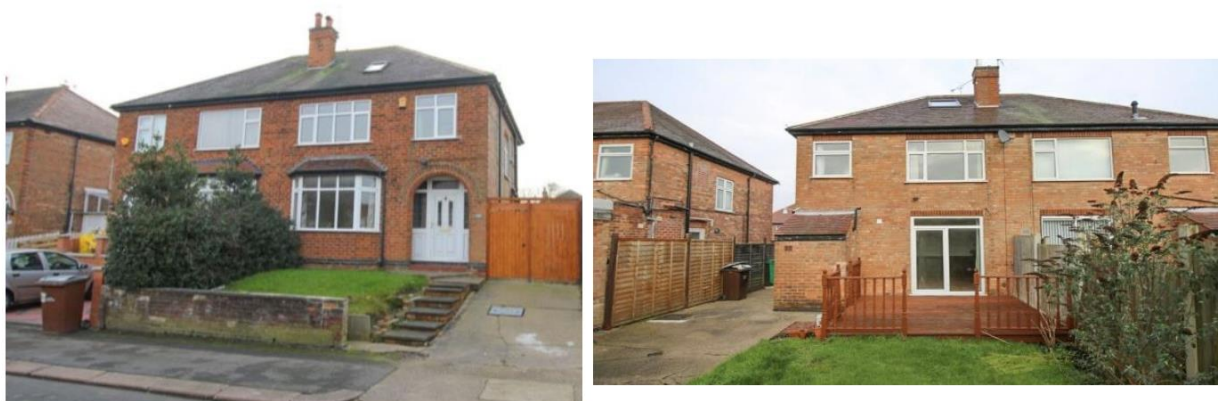
Figure 8 Front and rear photos of Nottingham house
