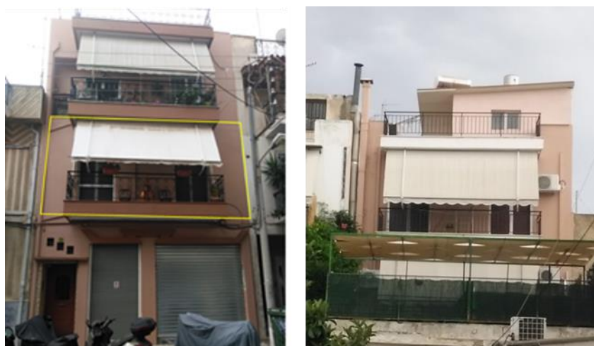
Figure 50 -The main (front) and backside façade of the building – the renovated apartment is indicated inside the yellow rectangle
