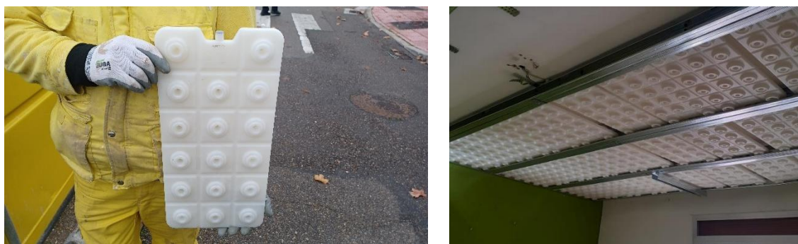
Figure 40 - Installation of PCM panels
