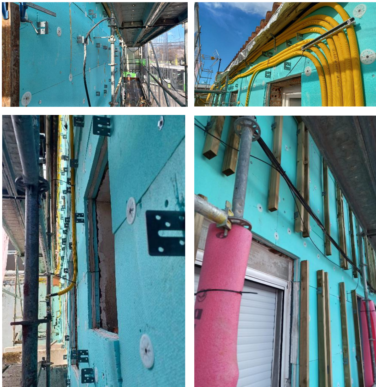
Figure 37 - Installation of prefabricated panel and rafters
