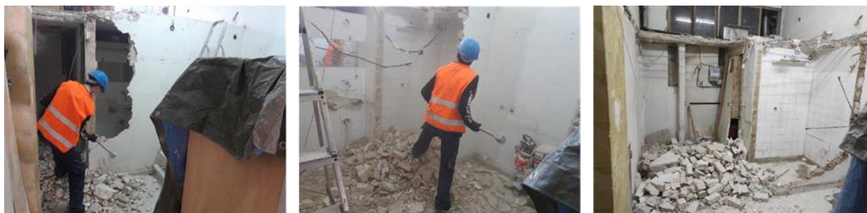
Figure 60 - Demolition of the wall on the ground floor where the water tank would be installed
