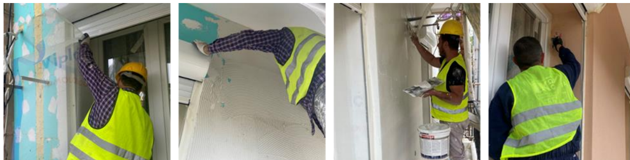
Figure 65 - Installation of the fiberglass mesh, applying the glue coatings, smoothing the surfaces, applying the final paint
