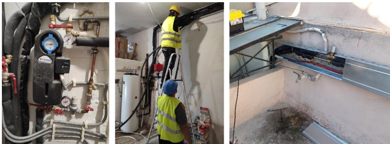
Figure 62 - Installation of piping and wiring of the PVT system
