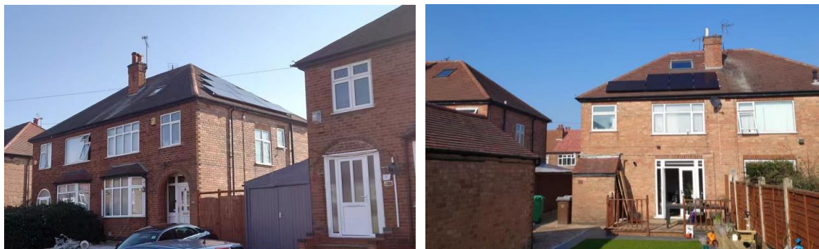
Figure 13 - PV panels installed on the west (Left) and south (Right) roof
