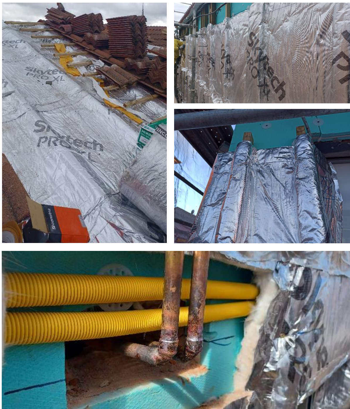
Figure 38 - Installation of the Winco rainscreen, reflective and airtightness membrane
