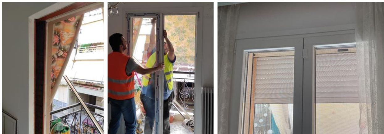
Figure 69 - Removal of old window and balcony doors and installation of new ones
