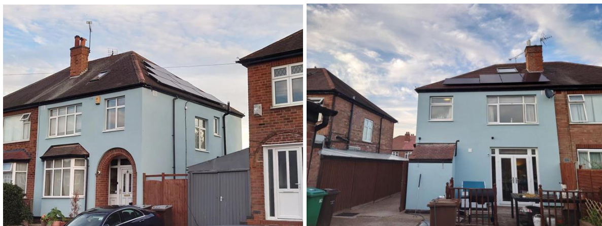
Figure 15 - External wall insulation and Solar PV Front (Left) and Back (Right)
