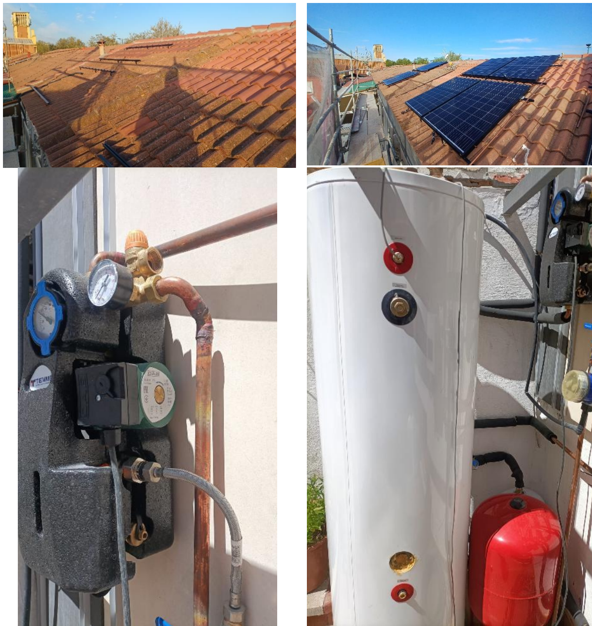
Figure 43 - Installation of the PV/T panels
