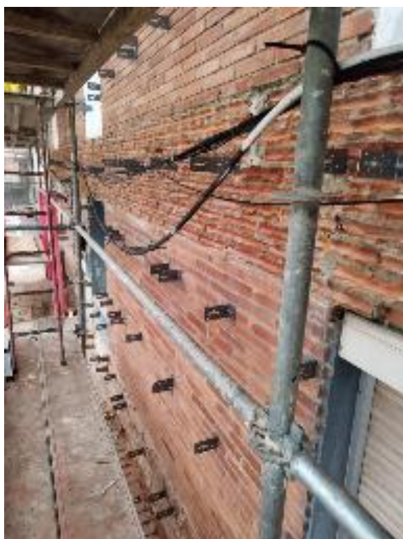
Figure 36 - Drafting and installation of anchors
