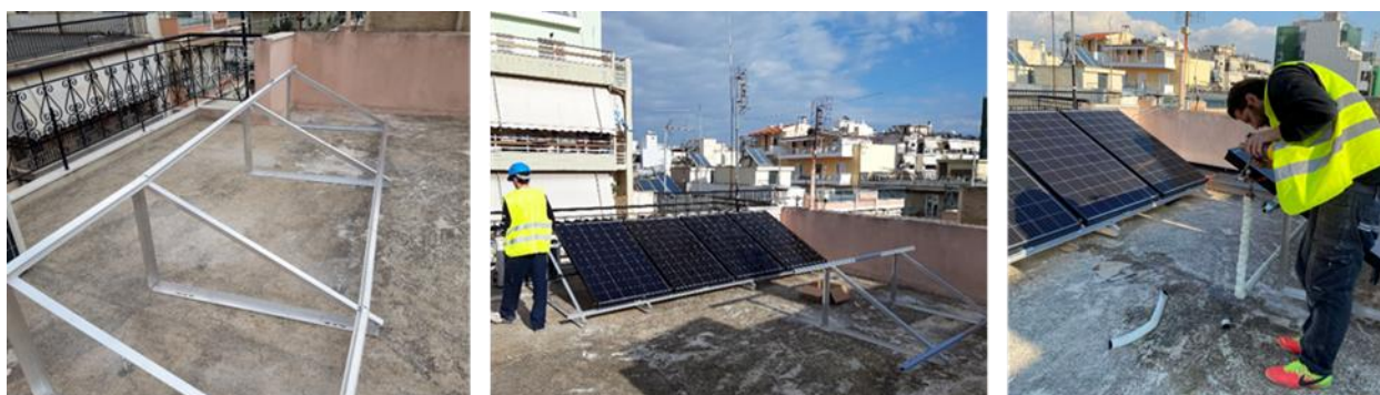
Figure 63 - Installation of the mounting system and of the photovoltaic panels of the PVT system
