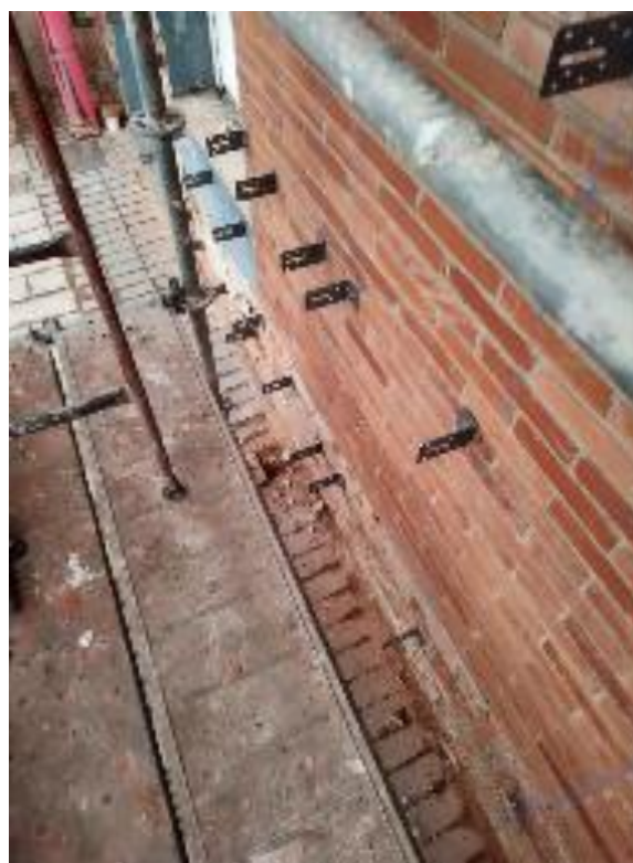
Figure 36 - Drafting and installation of anchors
