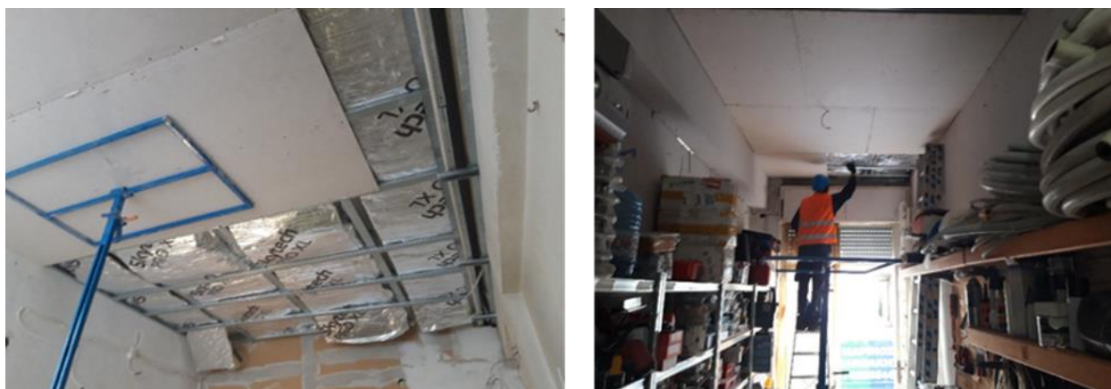
Figure 68 - Installation of false ceiling panels
