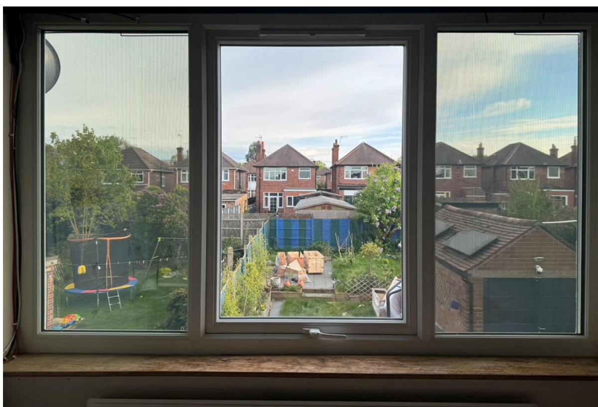
Figure 14 - Installation of the PV-Vacuum Glassing Windows unit
