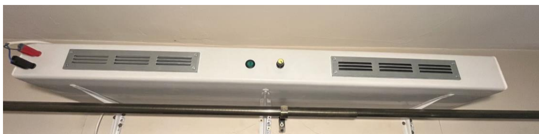
Figure 20 - Installation of the Window heat recovery inside the bedroom
