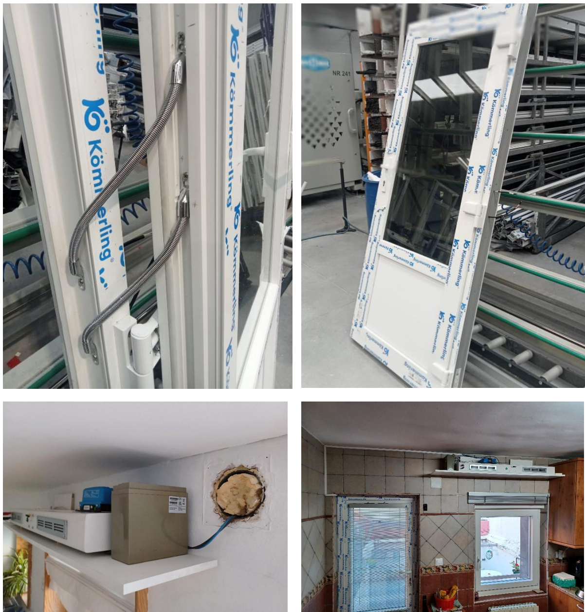
Figure 41 - Installation of the PV vacuum glazing window and the window heat recovery
