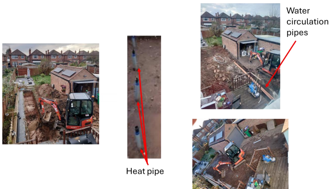
Figure 17 - Installation of the heat-pipe and water circulation pipes of the GSHP system underneath the soil
