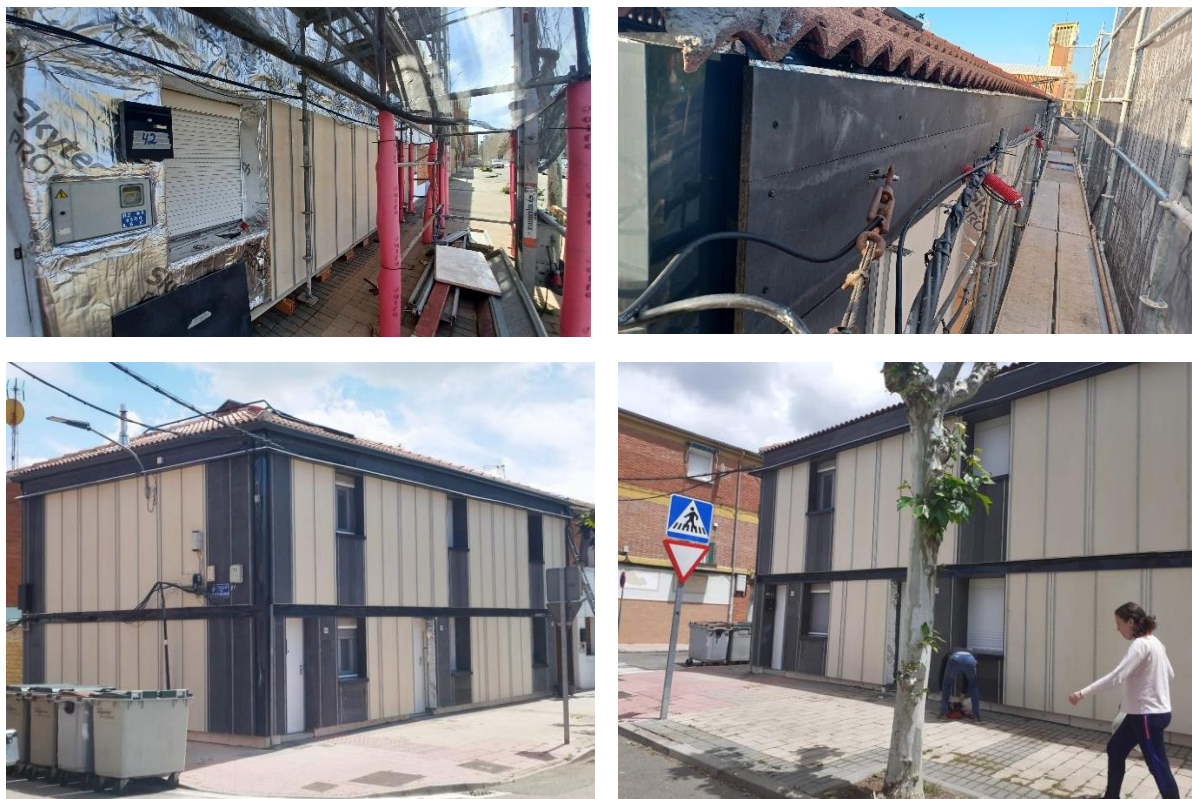
Figure 39 - Installation of the finishing boards
