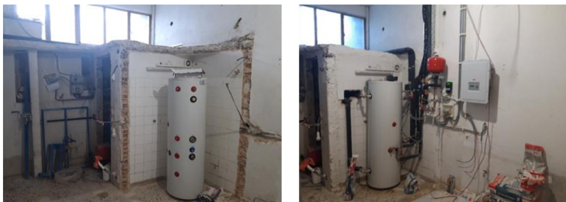
Figure 61 - Installation of the water tank and of the related auxiliary equipment
