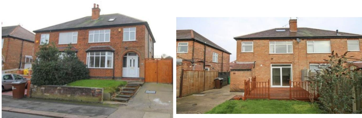
Figure 1 - Front and rear photos of Nottingham house
