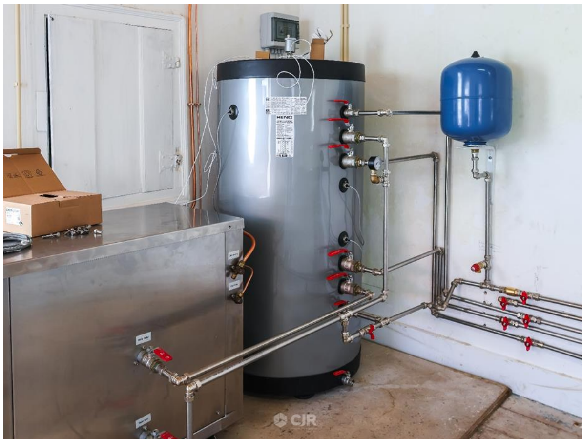
Figure 79 - Solar-Assisted Heat Pump - Portuguese demo case
