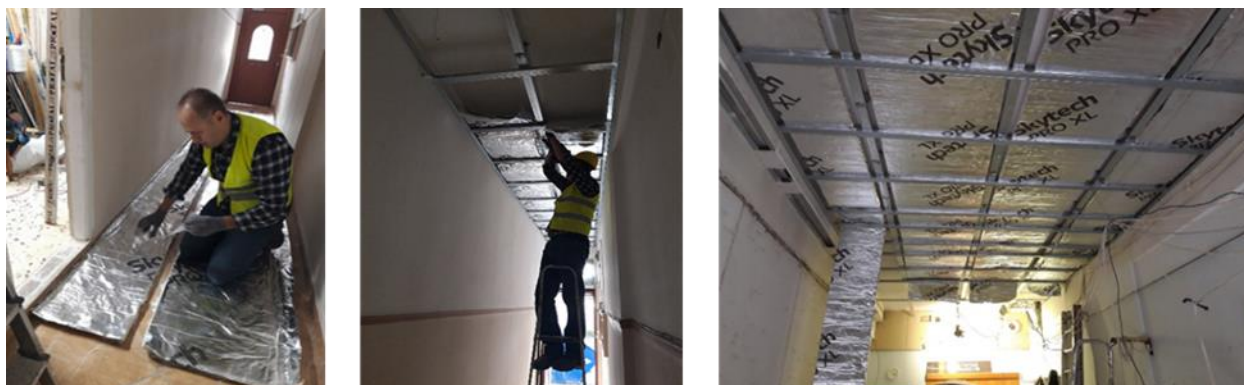
Figure 67 - Preparing the WINCO membrane and the new ceiling frame for the installation of the membrane
