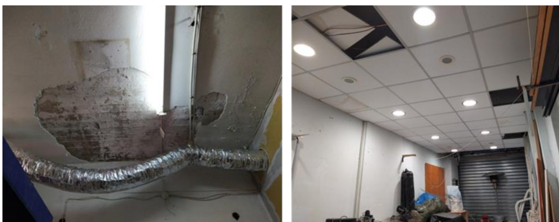
Figure 54 - The ceiling of the ground floor with which the demonstration apartment is in contact
